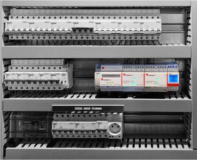
The system equipment, such as routers, power supplies, etc., has been reinstalled in the control cabinet.
